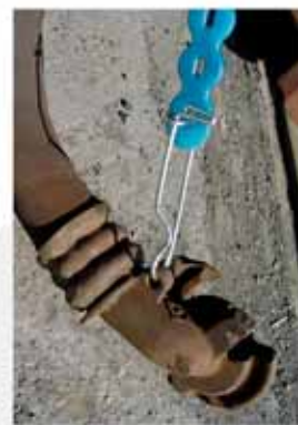
Polymer support with revised lower clip
